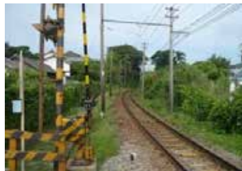
踏切・電路・軌道設備
